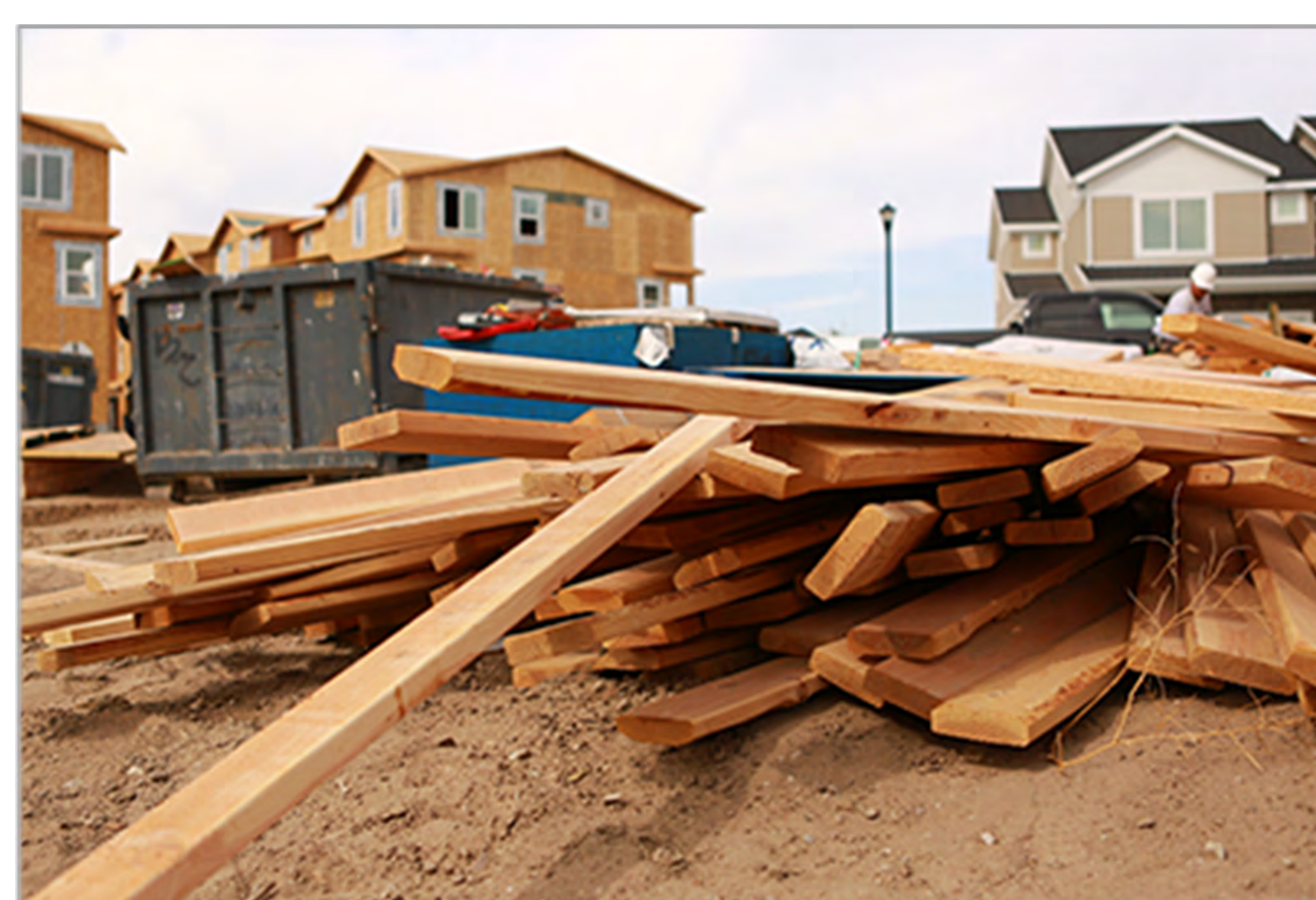
STICK FRAME JOBSITE
