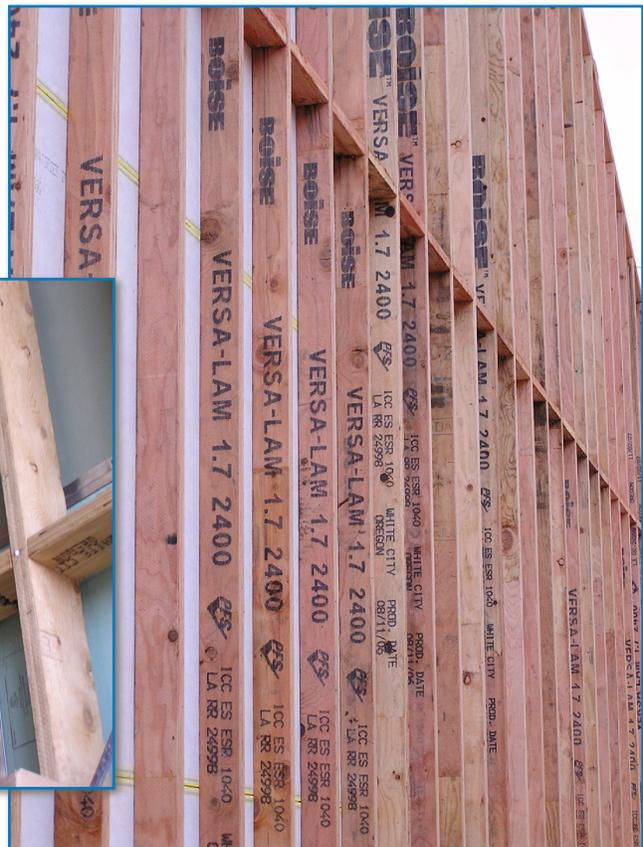
Deflection of individual wall studs is calculated similar to that of joists and beams. The stud height, on-center spacing and stiffness determine the deflection from a design wind load. Below are the building code deflection limit provisions dependent upon the wall coverings.
