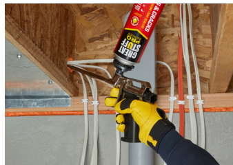
Electrical wire penetrations
