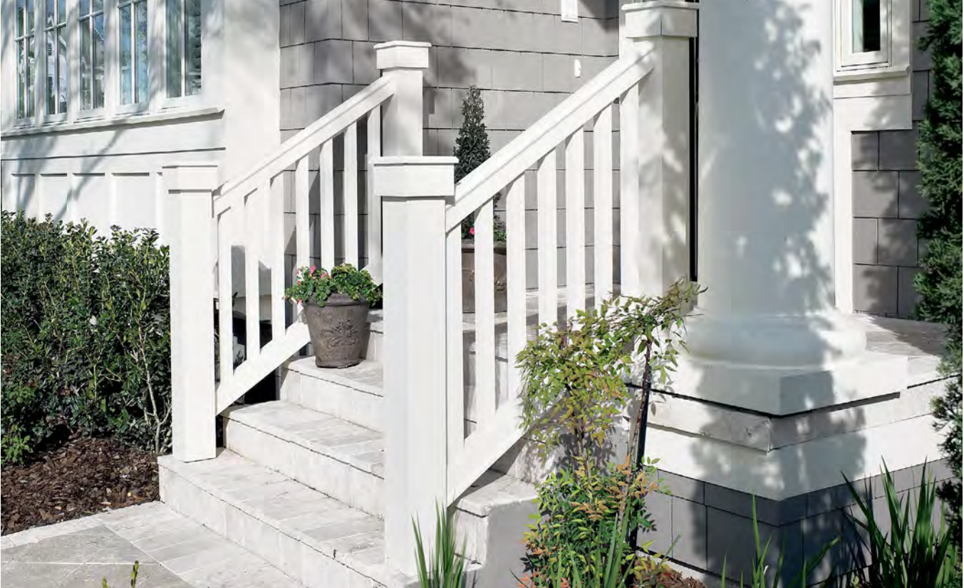
Note: Porch / deck surface pictured above was 30" or less above grade.
