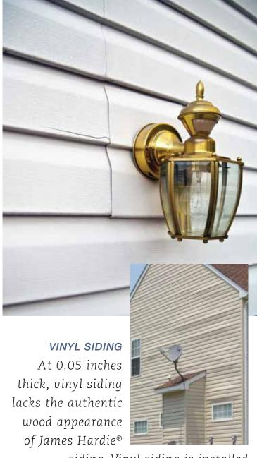
siding. Vinyl siding is installed in "panels" which create larger, more visible seams.
