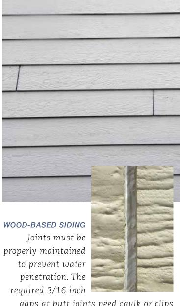
gaps at butt joints need caulk or clips which increasingly accentuate the gaps since they can fade at a different rate than the siding.
