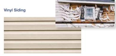
Vinyl siding is a plastic exterior that was introduced in the 1960s as an alternative to aluminum siding. While it certainly has plenty of merits in comparison to aluminum, vinyl siding comes with its own set of vulnerabilities: hail, the sun's UV rays, fire and heat can cause it to crack, buckle, warp-even melt.
