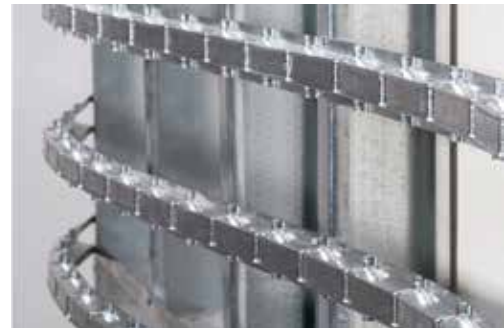
Typical Ready-Hat Installation
