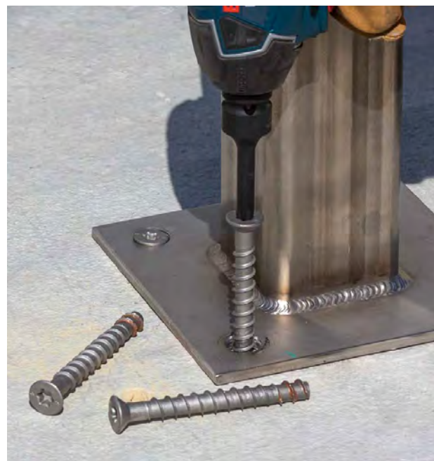
Titen HD Countersunk Installation
