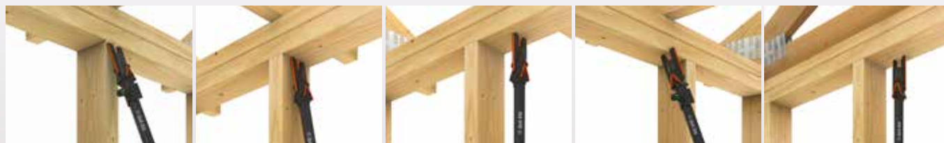
Narrow face of stud location.
