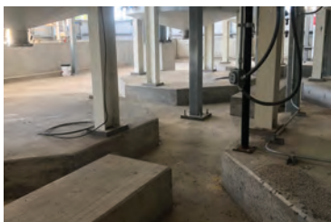
Typical medium-corrosive environment — exterior anchorage.
