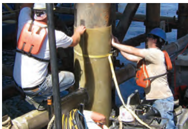
FX-70® structural piling repair and protection system
