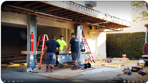
Bessemer Soft-Story Retrofit Case Study
